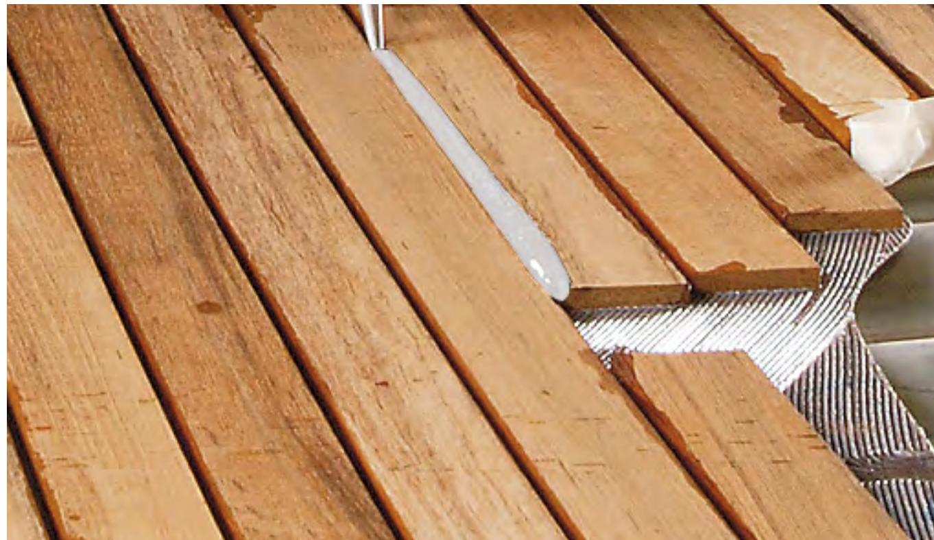
With dispersion adhesives, for example, ship decks made of wood are glued. In this case, the water resistance of the adhesive is required.
